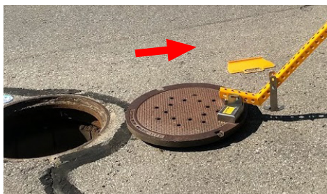
Slide cover away from manhole
