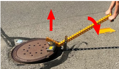
Slide cover away from manhole
